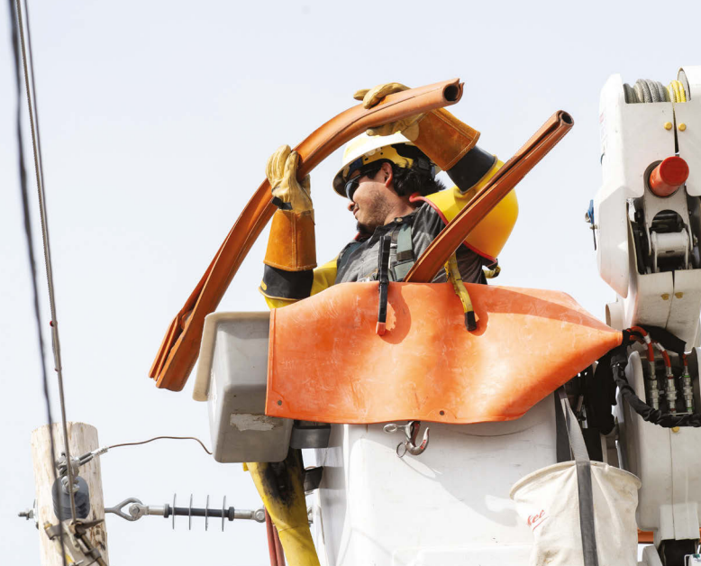
Left: Andy Garcia puts cover-up materials on the hot line he will be working on. He is a third-year apprentice and can work energized lines as long as he is supervised by a journeyman lineman. Right: Briar and Andy knock dirt off the auger as the hole for a replacement pole is dug. Apprentice linemen do a lot of the grunt work for electric cooperatives. They will need 8,000 hours of on-the-job training to advance to journeymen.
