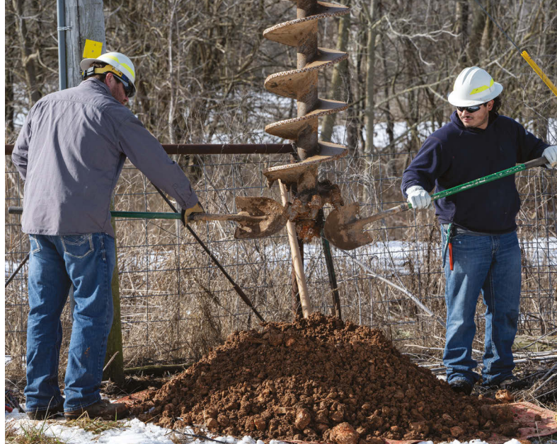
Left: Andy Garcia puts cover-up materials on the hot line he will be working on. He is a third-year apprentice and can work energized lines as long as he is supervised by a journeyman lineman. Right: Briar and Andy knock dirt off the auger as the hole for a replacement pole is dug. Apprentice linemen do a lot of the grunt work for electric cooperatives. They will need 8,000 hours of on-the-job training to advance to journeymen.
